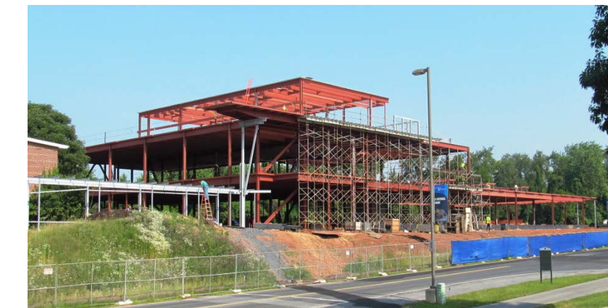
Building Structural Frame
