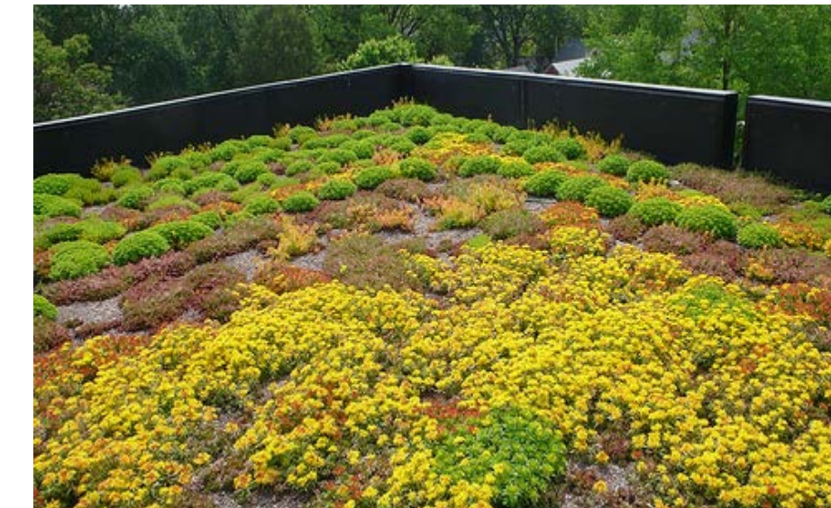
Extensive Green Roof System
